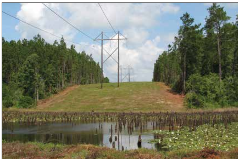
Great River Energy heavily invests in a vegetation management program. Identifying vulnerabilities and keeping trees clear of the lines helps ensure that branches don’t hit or fall onto power lines, causing damage and knocking out the electricity.
