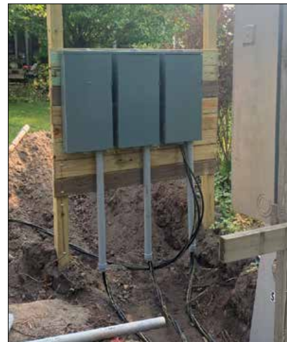
(top) All three panels needed to be replaced. (below) New cabling.
