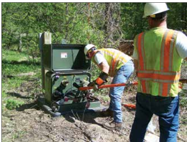
Pad mounted transformer, photo courtesy of Runestone Electric Association
